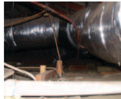
Example of access limitations in roof void.
